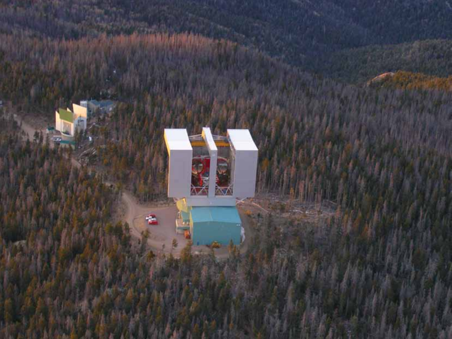
The LBT is on the summit of Mt. Graham showing the 30-m high shutters open and the two 8.4-m mirrors looking out. The white enclosure is fully rotatable. At left is the Heinrich Hertz 10-m submillimeter radio telescope. This view was taken from a helicopter.
